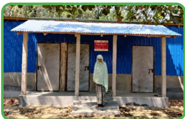
Rebuilding hope — new houses constructed for families who lost their homes in Cyclone Mocha.
