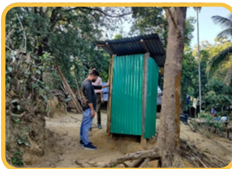
Building sanitation, restoring dignity — PHALS supports families with new latrines.
